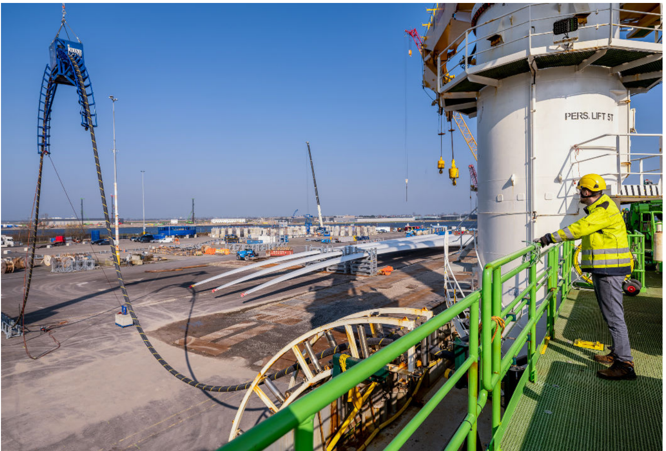
Loading a subsea cable onto the Viking Neptun in Amsterdam. This cable was used for installation at the Dogger Bank Wind Farm, UK
