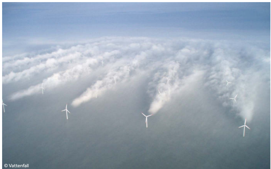
Horns Rev 1: Innovative technology to understand the health status of the last generation turbines, and to know when to administer preventative or protective measures, is the cornerstone of reducing the operational cost
