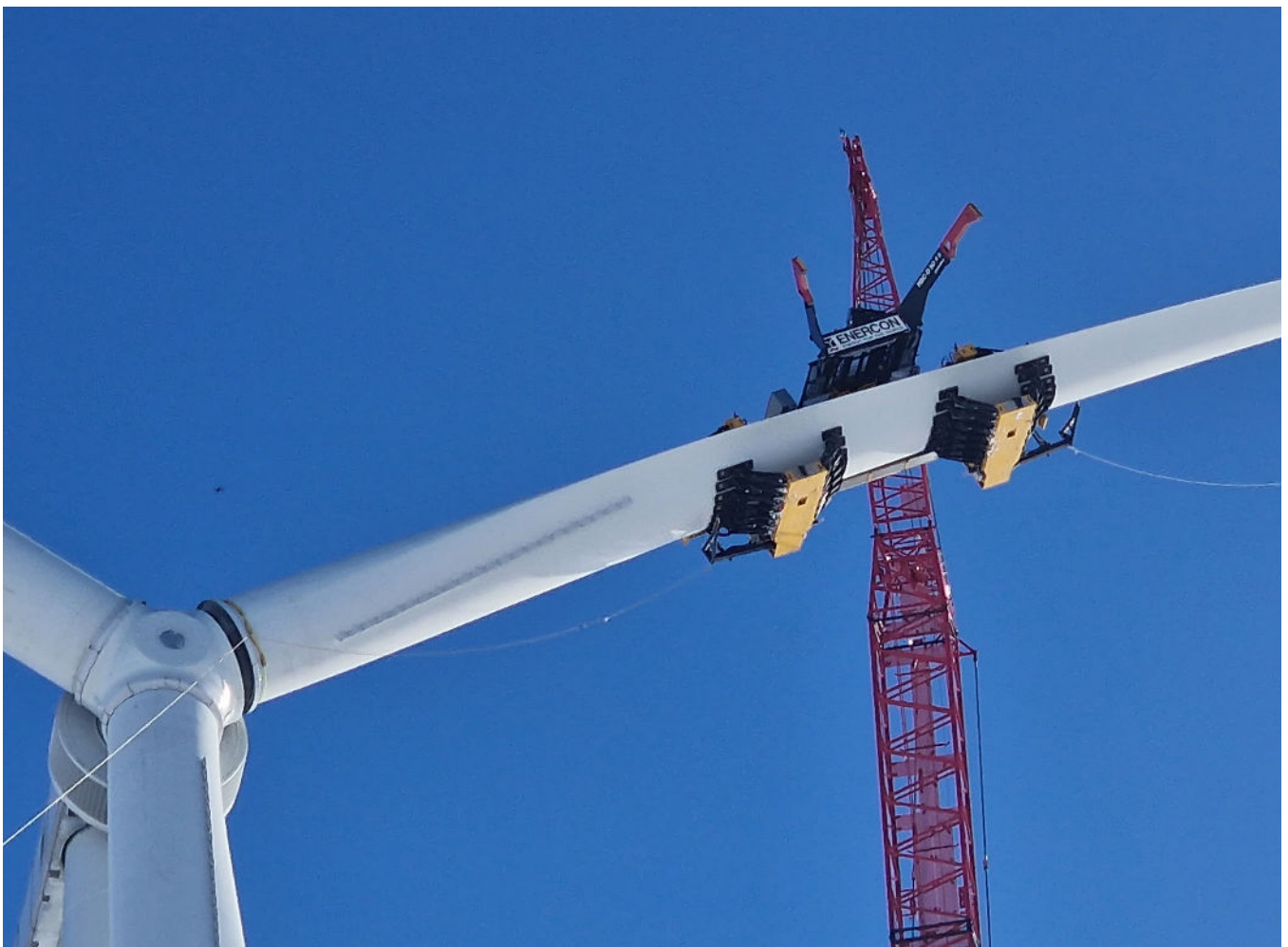
With its RBC-D yokes, ematec has revolutionised the assembly of rotor blades
