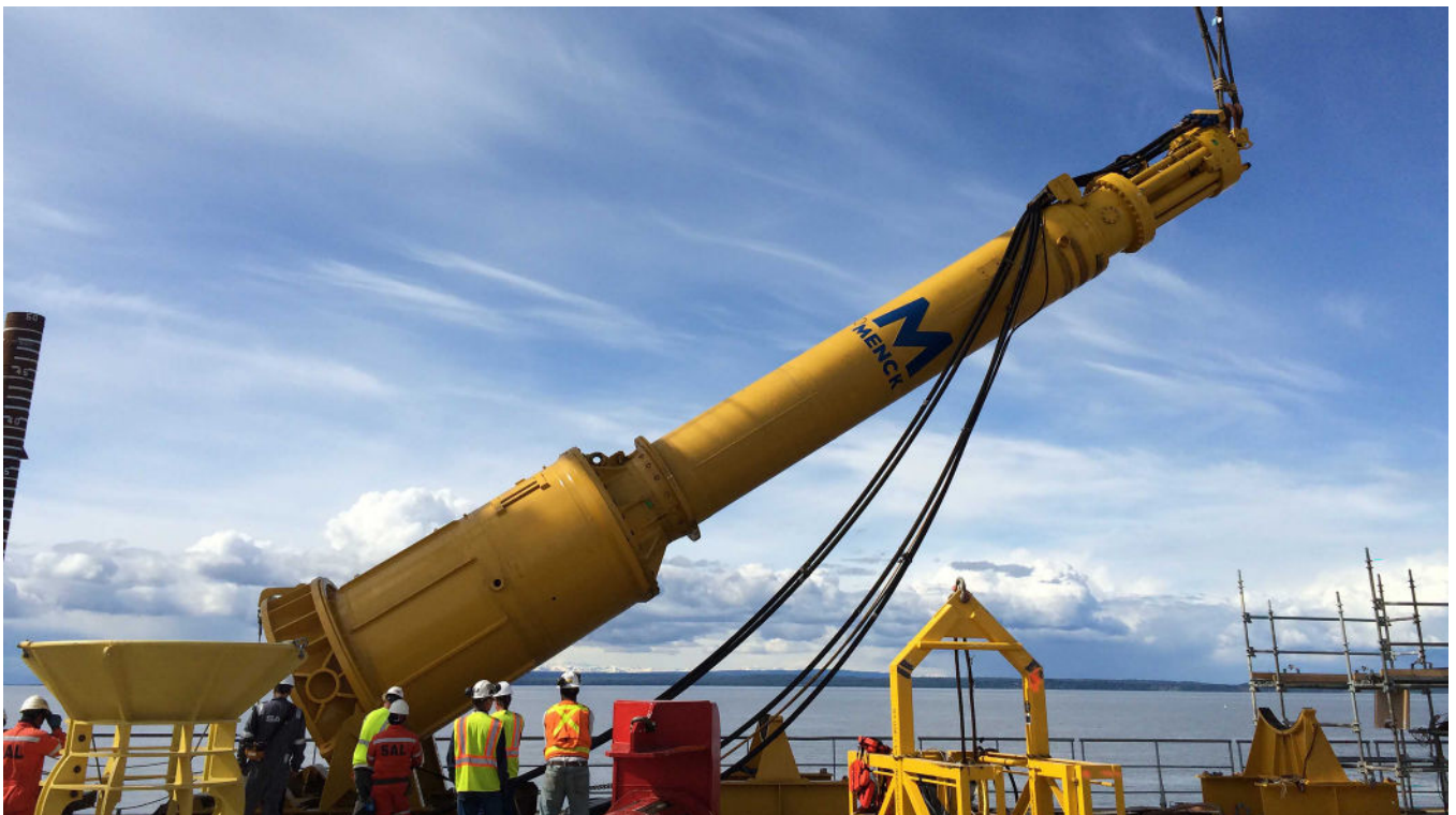
Hammer configuration for deep water installation
