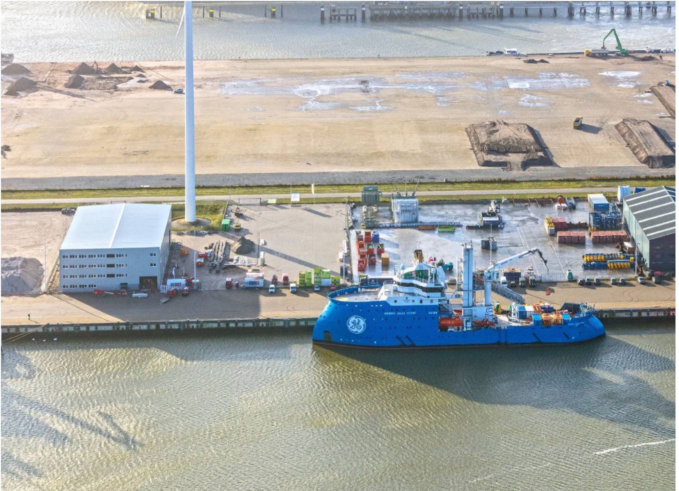
CPS Eemshaven Facility
