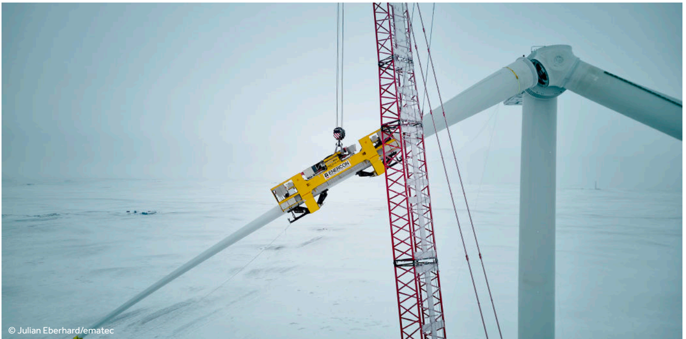
The RBC-D50 rotor blade yoke from ematec is in use worldwide
