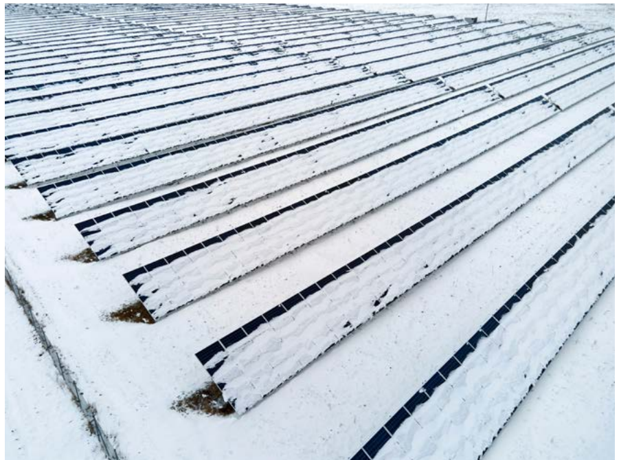
In some areas, snow can remain on the modules for months, threatening the profitability of the project
