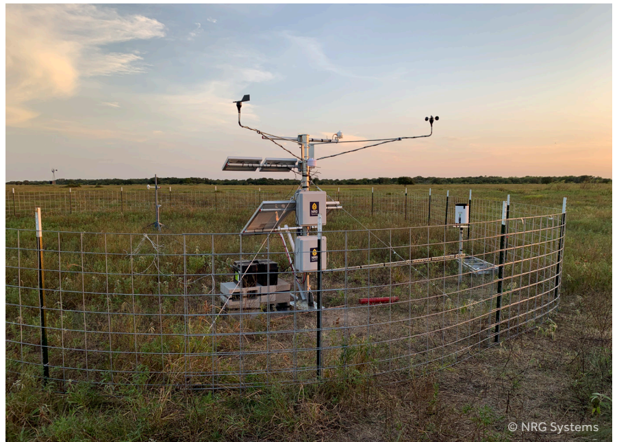
Example Solar Resource Assessment (SRA) station installed on-site
