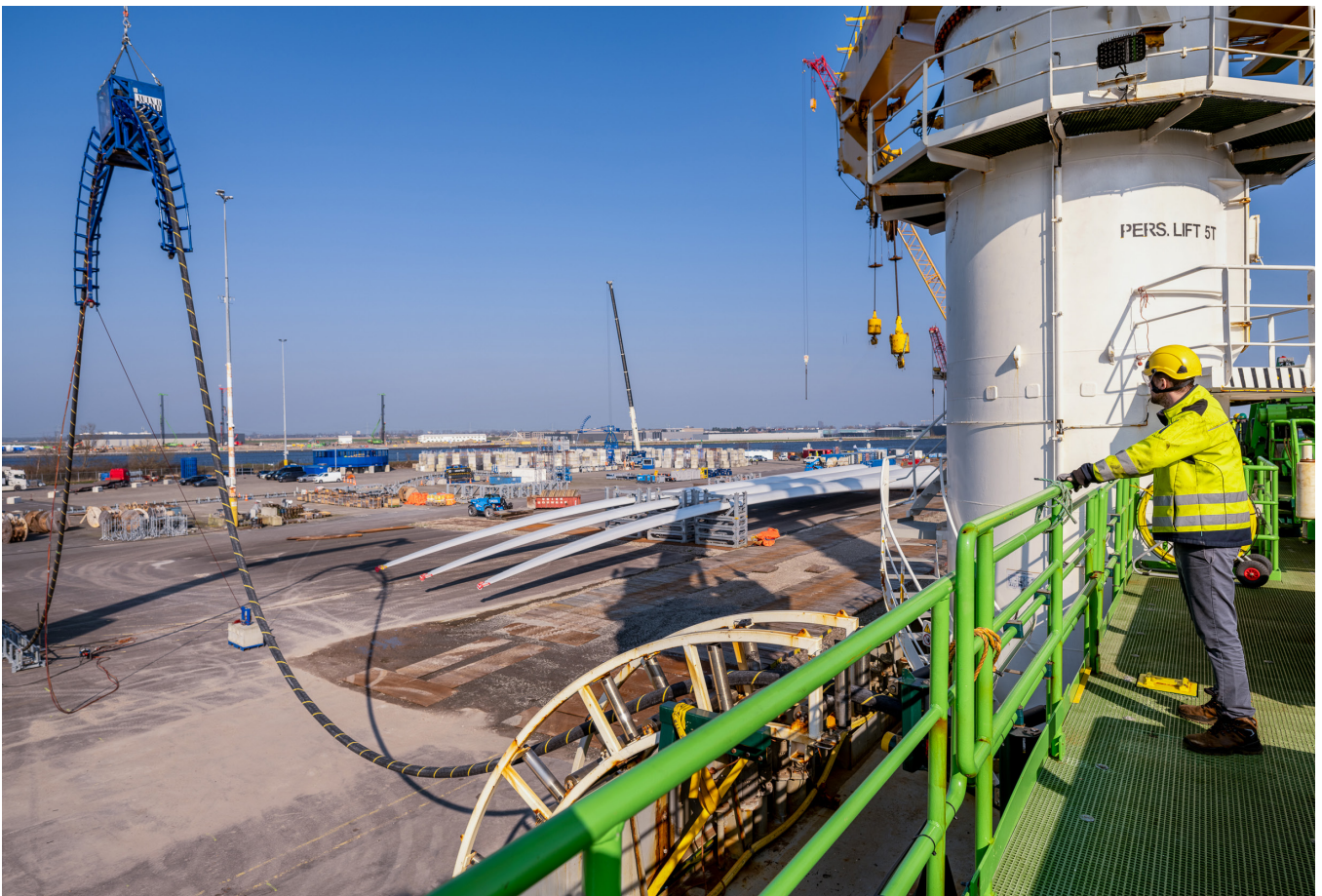
Loading a subsea cable onto the Viking Neptun in Amsterdam. This cable was used for installation at the Dogger Bank Wind Farm, UK
