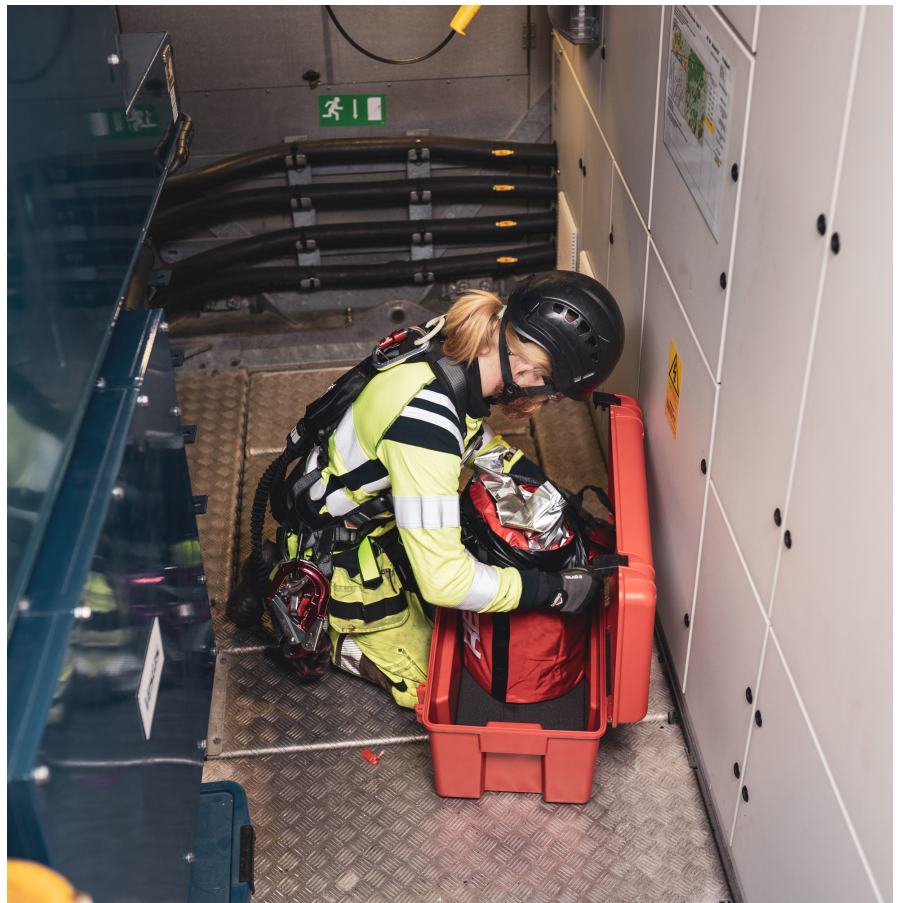
Red Box: storing turbine evacuation solutions within the nacelle
