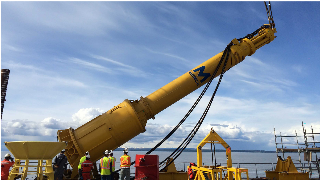
Hammer configuration for deep water installation
