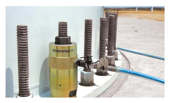
use and extremely efficient in their speed of operation. Torquing is used on tower segment bolt connections as well, not just tensioning. The square drive torque wrenches tend to be used.
