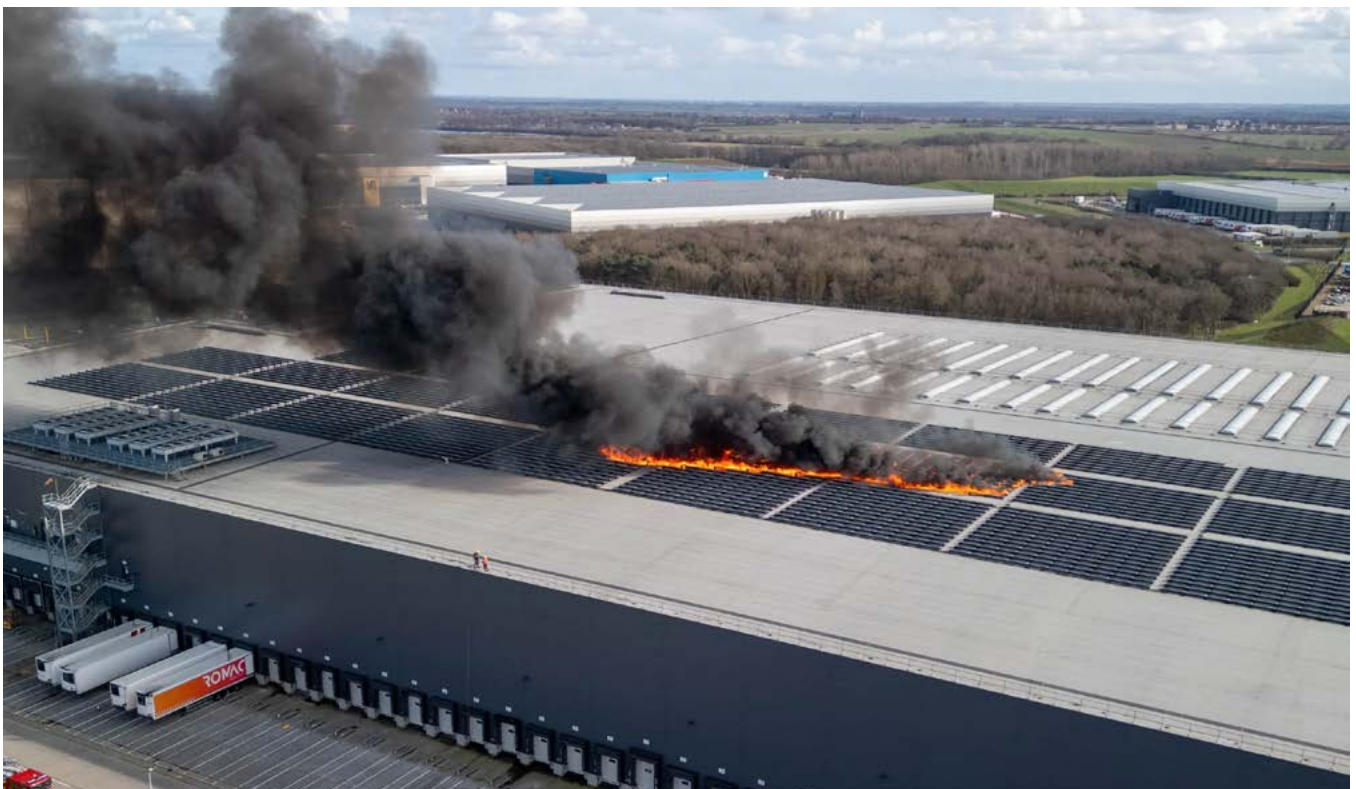
Figure 5: Solar panels catch fire at Lidl distribution centre in Peterborough. Arguably it is possible to avoid such events by a combination of rational system design, component quality, craftsmanship and preventive troubleshooting
