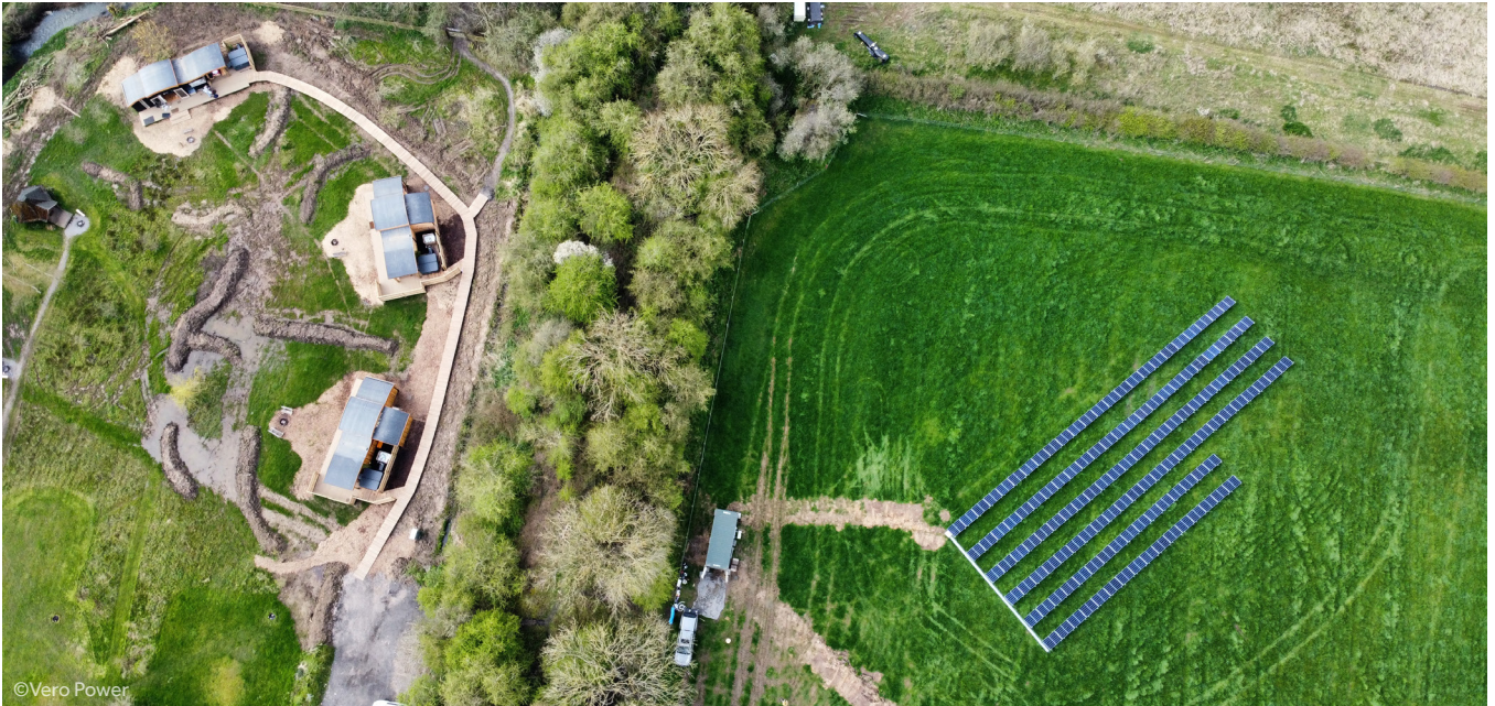
52 kW PV system and 120 kWh energy storage with BYD Battery-Box systems
