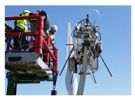
the turbine blade. However, due to operational restrictions imposed by regulatory legislation, commercial drones are not yet fully matured and commercially available for such heavy lifting tasks. Therefore, until heavy lift drones become more advanced and widely accessible, the company will continue to rely on traditional methods such as helicopters, cherry pickers, or cranes to bring the robot onto the blade.
