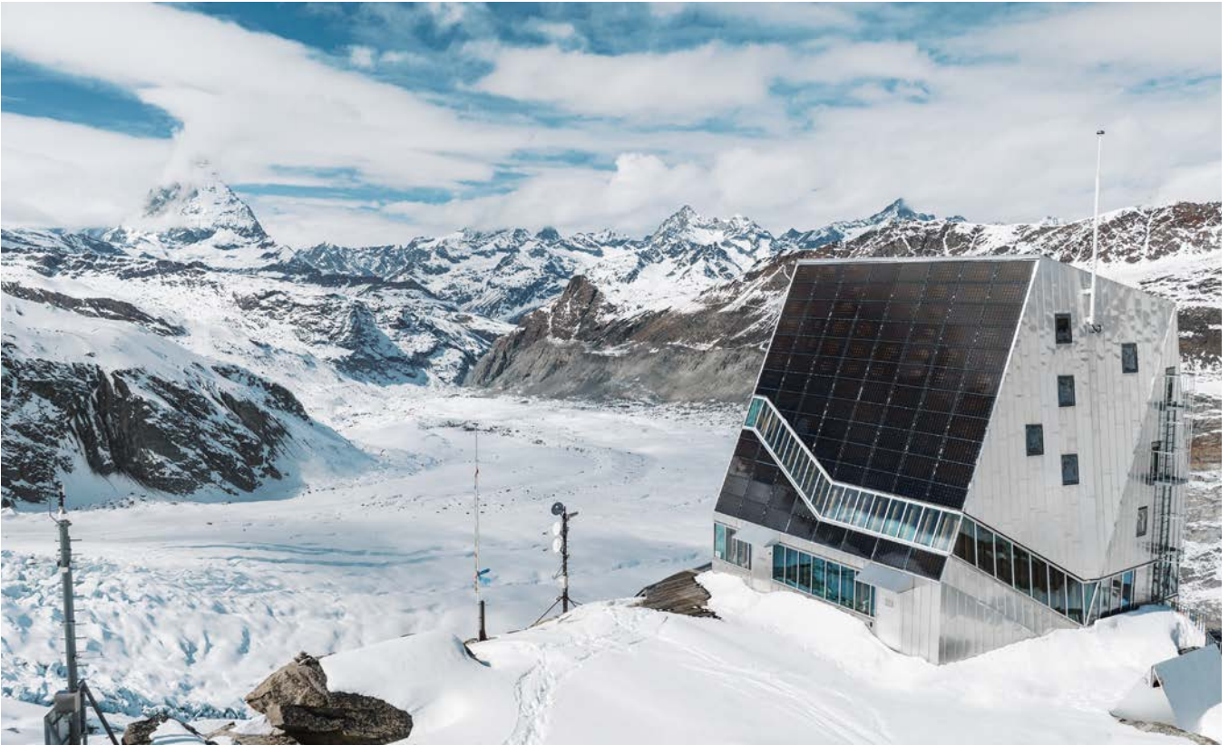
Building integrated PV installation at alpine resort Monte Rosa in Zermatt/Switzerland at 2883 m. asl
