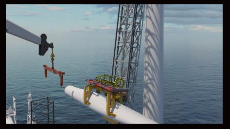
The WBI vessel is also equipped with a knuckle boom crane. This proven technology picks up individual blades from the rack using a blade-handling tool designed by Danish blade-installation tool specialist Liftra. The tool ensures safe handling of the blades during installation to maintain their structural integrity for a 15 to 20 year service life.
