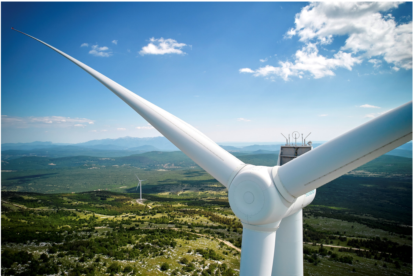
Figure 7: Commissioning of the first prototype by the wind energy experts from Phoenix Contact
