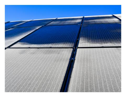
pyranometer, owing to radiative cooling at night and can lead to measurement errors, particularly early in the morning. Class A monitoring solutions compliant with IEC 61724-1:2021 are required to suppress dew and frost deposition, to ensure accuracy.
