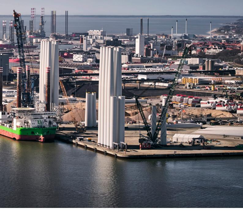
Consider the current plans for offshore wind in Europe, where the size of many offshore wind farms will exceed 1 GW, while components for the wind turbines continue to increase in size. Such projects will require storage areas of up to 50 hectares, and given the efficiency of the installation, the project campaign will be shorter than previously seen in offshore wind projects.
