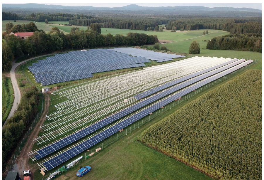
Figure 2 Installation of a PV power plant
