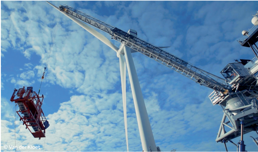
With its wide range of motion compensated gangway systems, Ampelmann is able to support floating blade maintenance and repair campaigns
