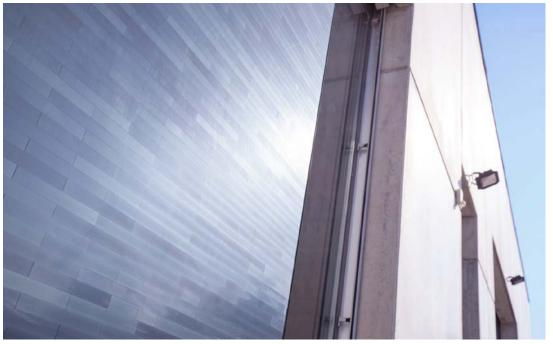
Matrix shingle modules are particularly suitable for integration into building facades with their high surface utilization, excellent performance under partial shading and aesthetic appearance. © M10 Industries AG
