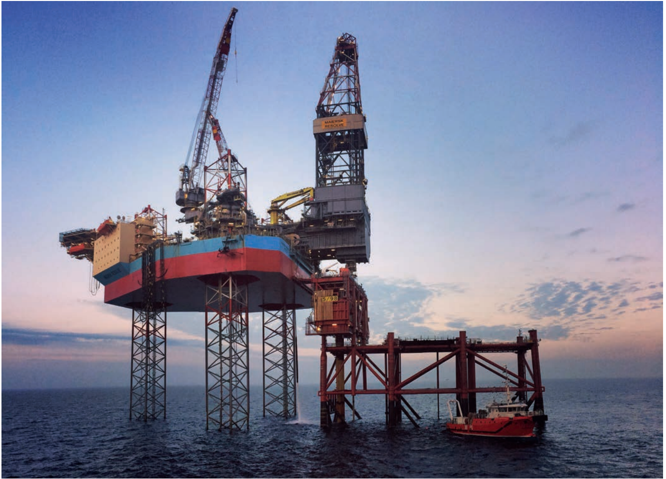
North Sea platform using solar electricity with Morningstar controllers to power telecom, navigation aid, bird deterrence, foghorn, and other critical systems. Courtesy JCE Energy
