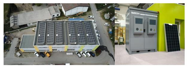
In December 2014 the company invested in a rooftop photovoltaic installation dedicated to self-consumption. Over the years, 20% of the production of the solar installation was consumed on site and 80% was injected into the public grid.
