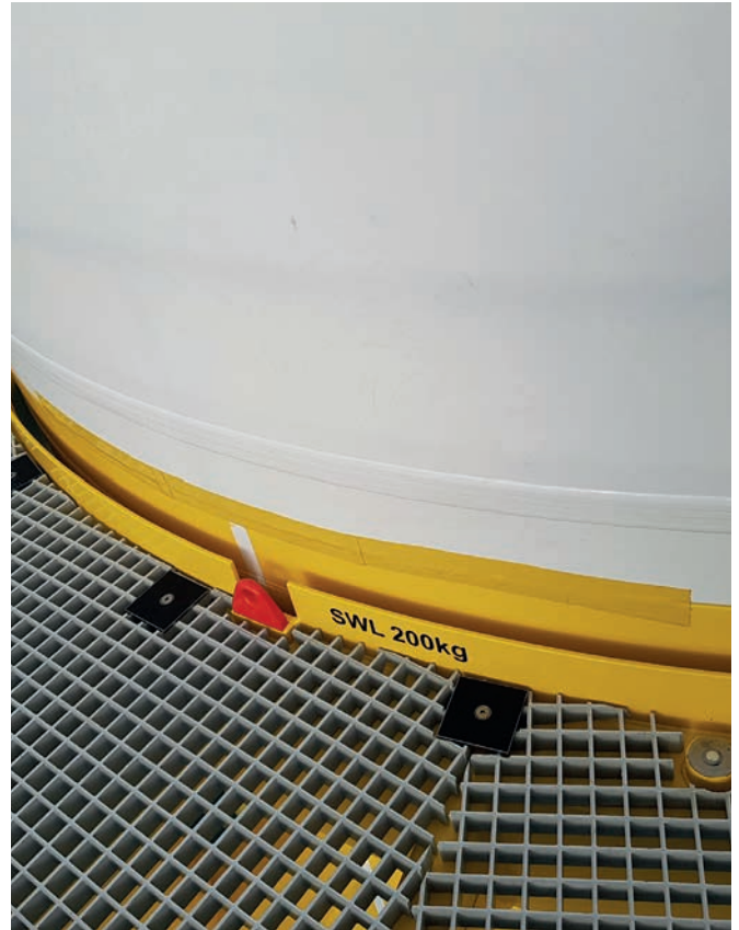
Offshore coating repair basecoat and self-cleaning patch
