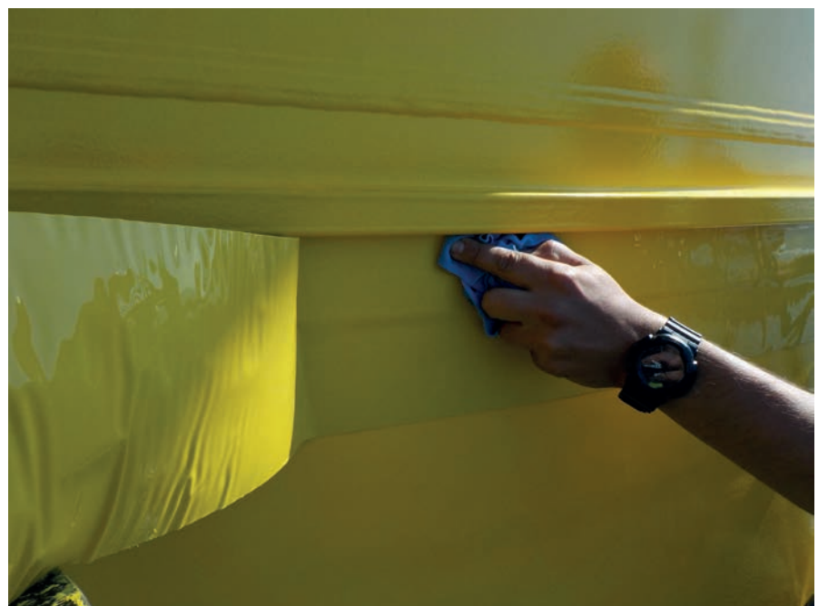
Close up patch replacement
