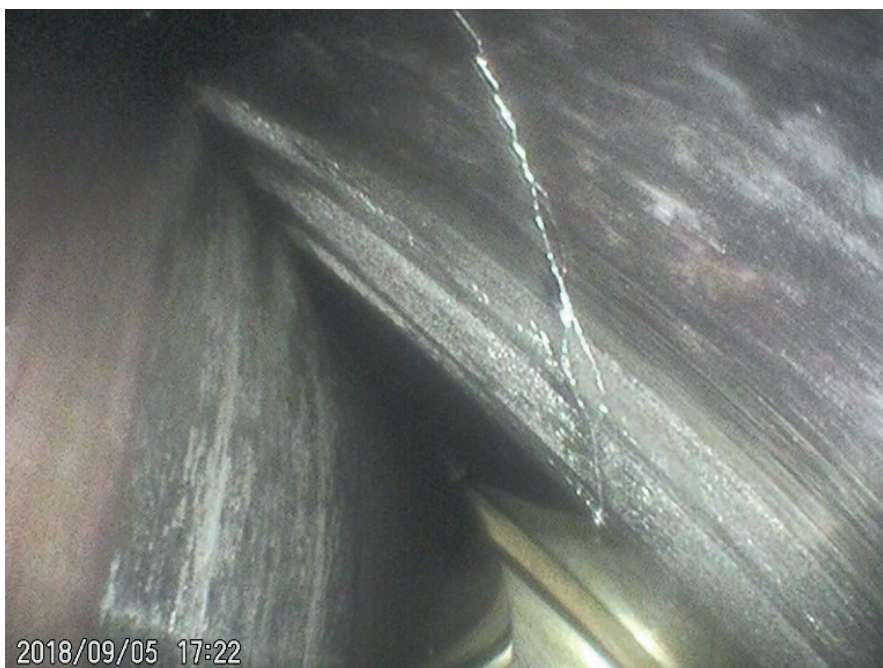
Figure 4: Known frequency components can give data analysis information supporting damage to the mechanical components. The image reveals an outer race crack on a bearing
