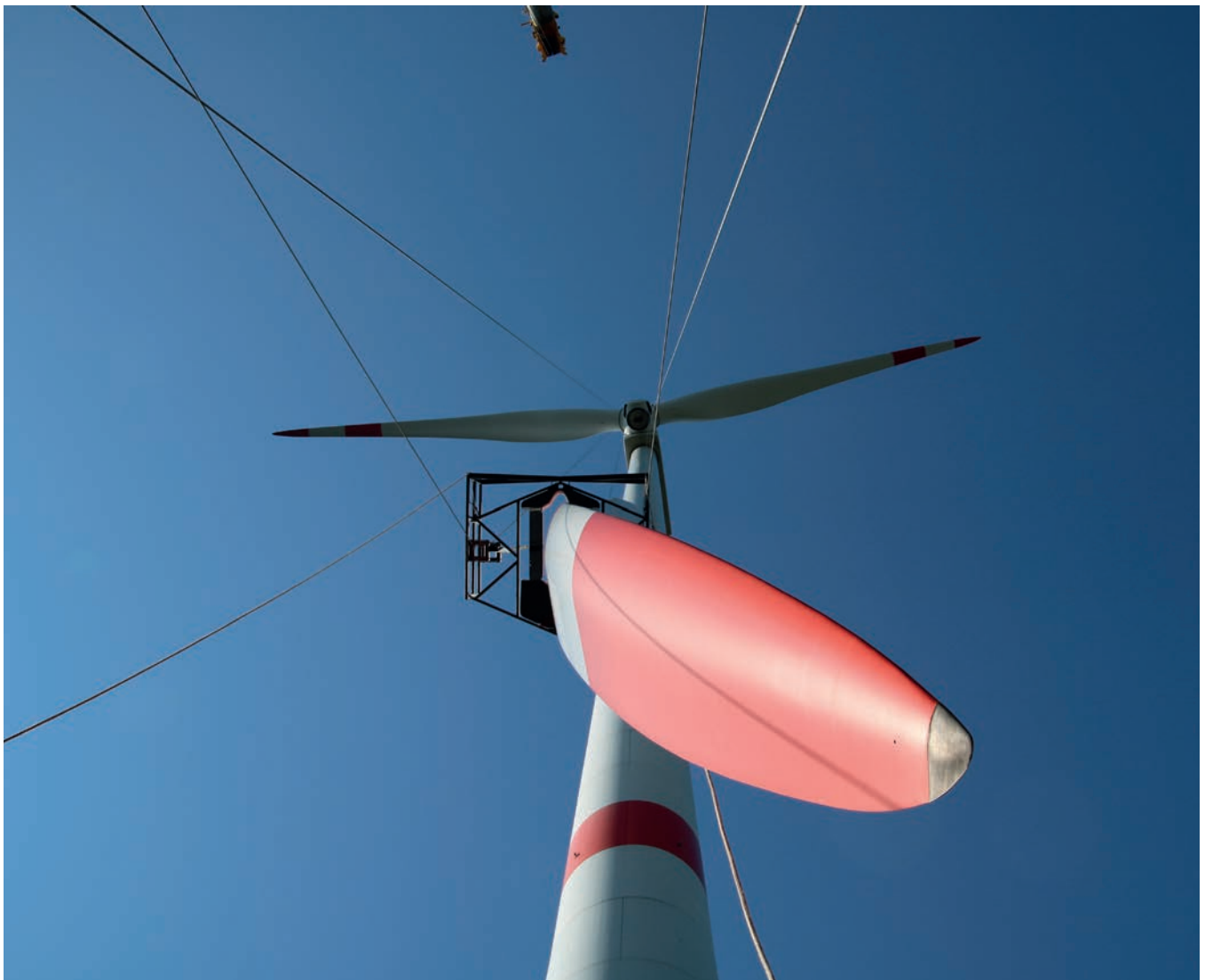
The rotor blade is lowered safely using clamping beams and winches
