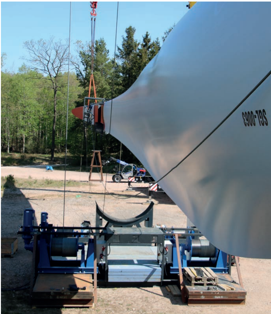
The rotor blade is safely placed on the blade support using the GBWS
