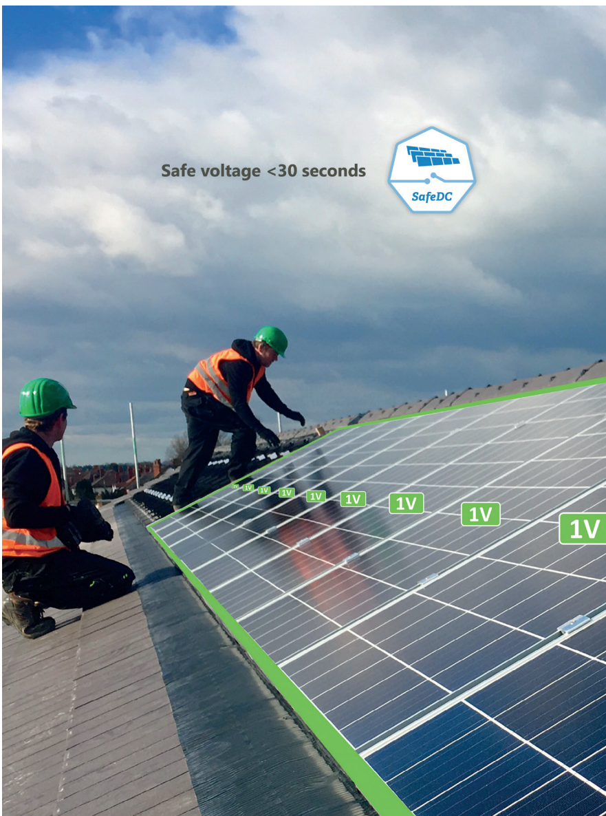
Roof SolarEdge SafeDC
