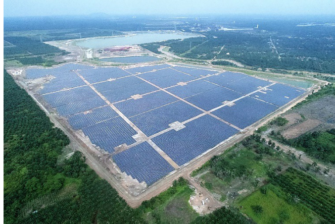
Above: TRe's large scale solar (LSS) farm in Sepang, Selangor in Malaysia
