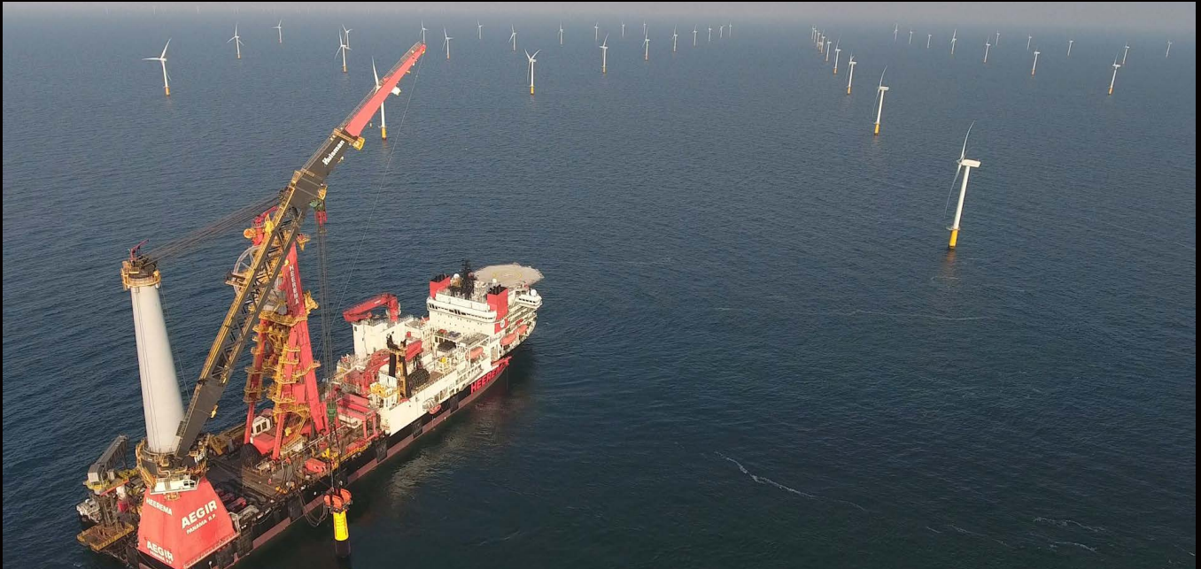
SJOR Monopile vibrated free hanging to final penetration Source: DOT
