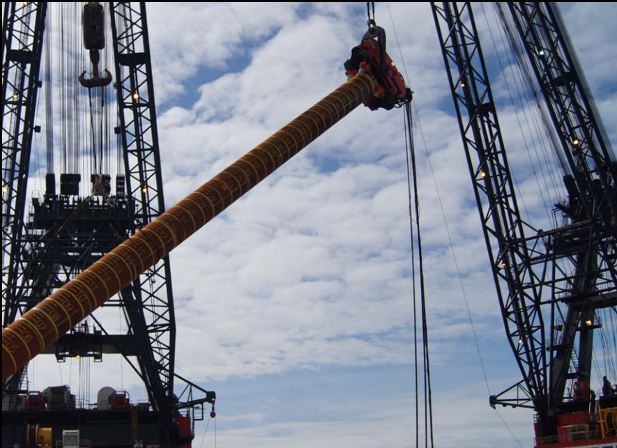
Dual crane upending of a 250t pile
