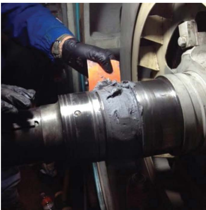
Belzona shaft repair
