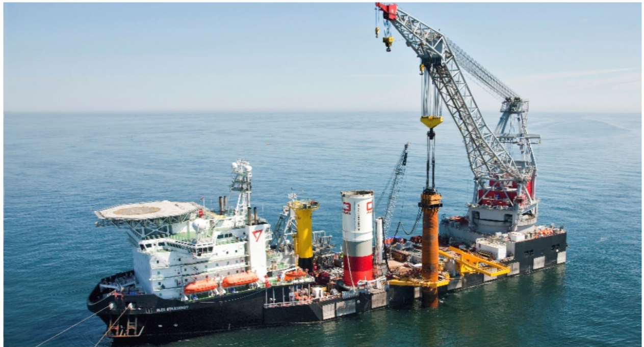
Picture 2: First deployment of a multiple vibro hammer for monopiles in 2012 at Riffgat OWF
