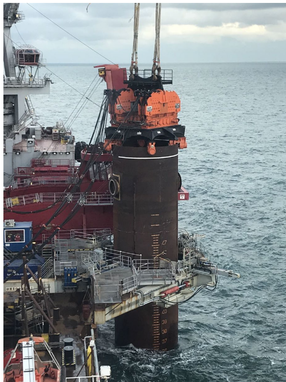
Picture 1: CAPE Holland's Vibro Lifting Tool driving a monopile for testing Seaway 7's motion compensated gripper
