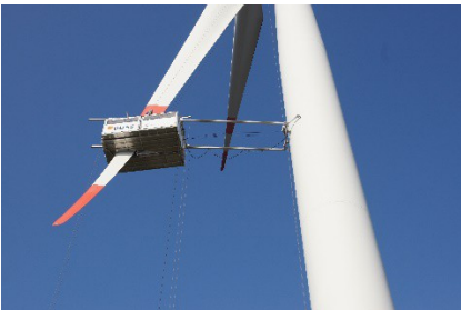
SYSTEM terra in operation ©WINDEA Offshore
