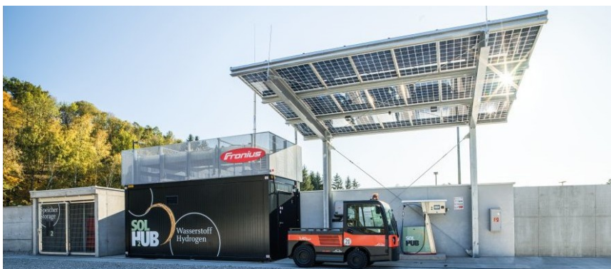
Fronius Solhub: Complete turnkey solution for decentralised solar hydrogen production, storage and refuelling of vehicles such as buses, lorries, working vehicles and special vehicles
