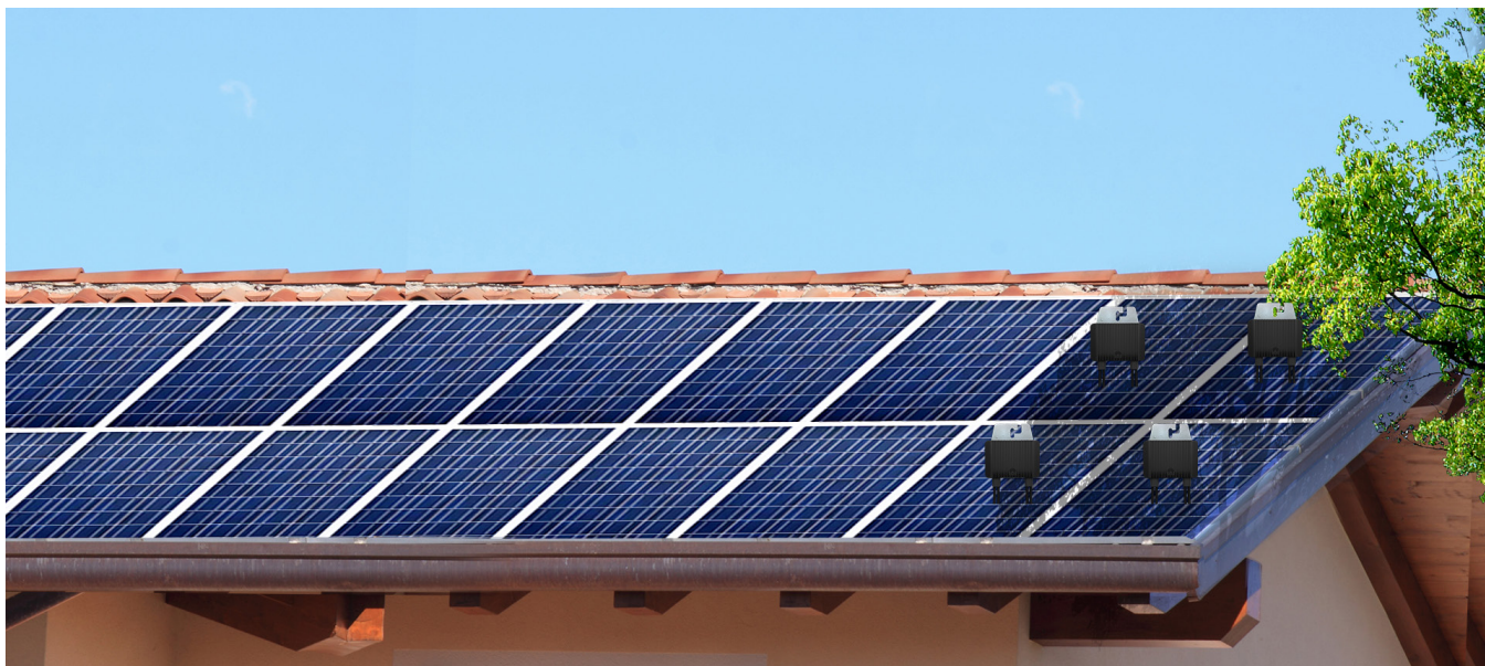
Illustration of PV layout with optimisers installed only on modules affected by shade.
