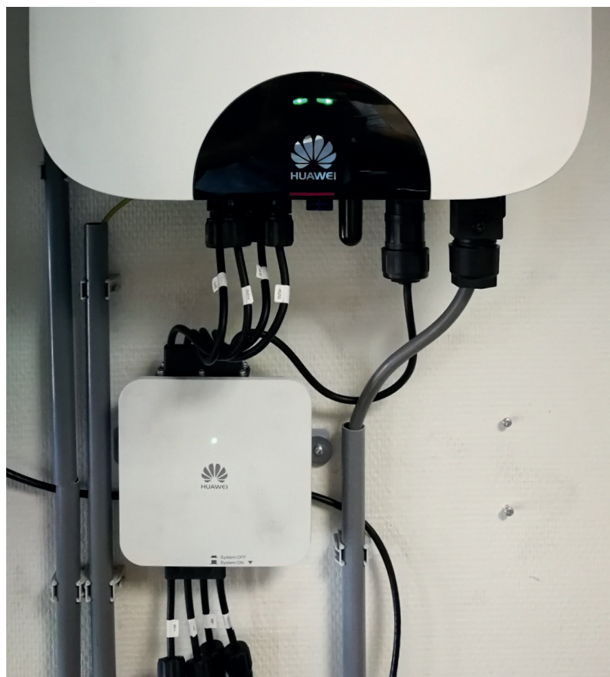
FusionHome SUN2000L Inverter and Smart PV Safety Box
