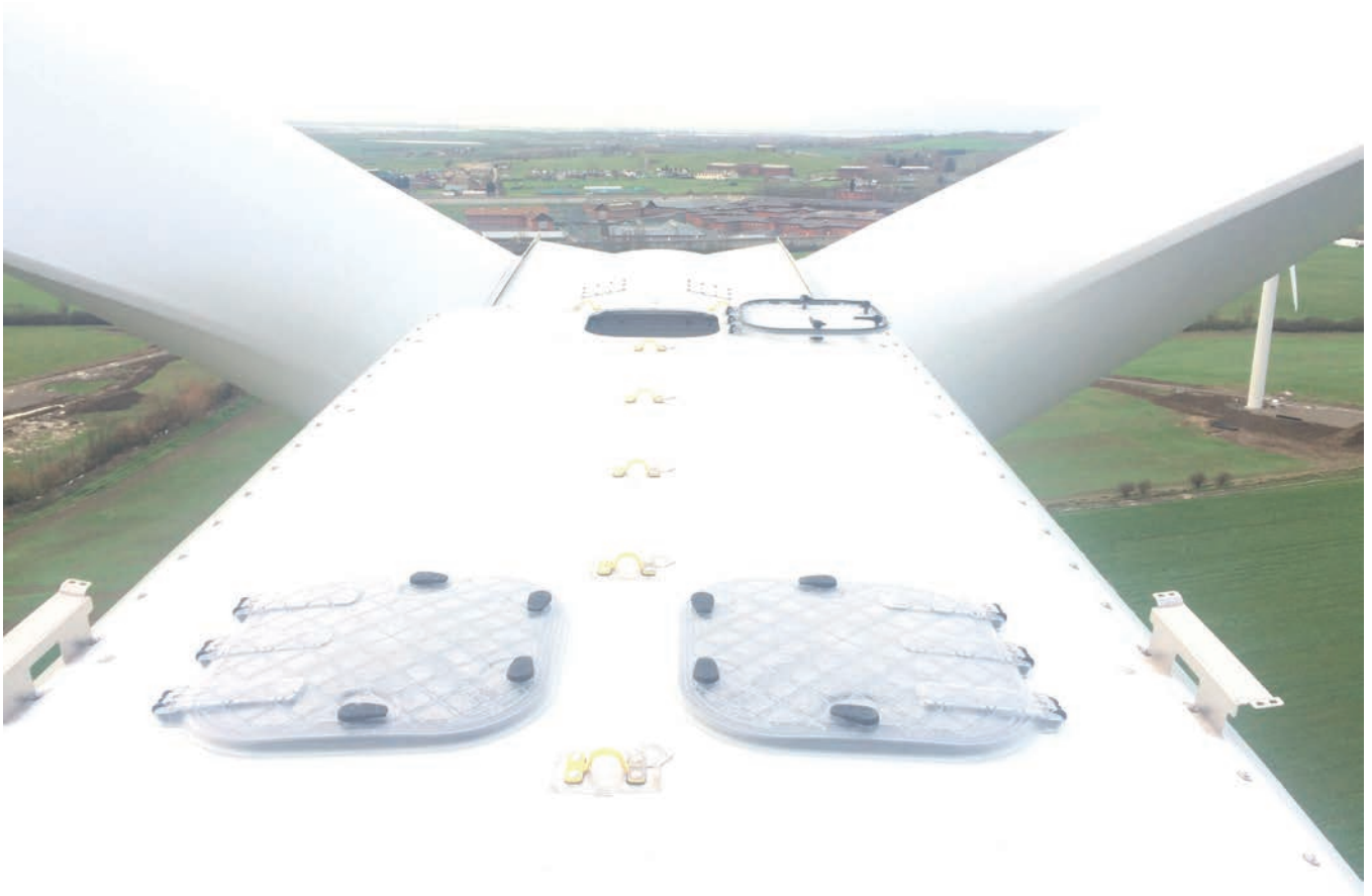
View over the rotor through turbine blades
