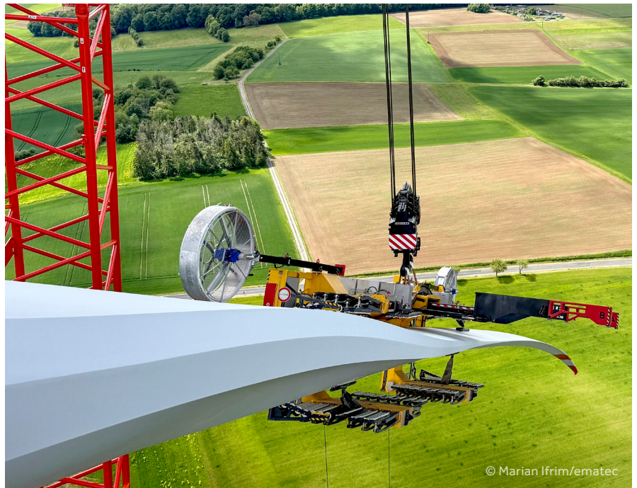
The RBC-D is designed for handling large rotor blades, including those used on 7 MW turbine platforms
