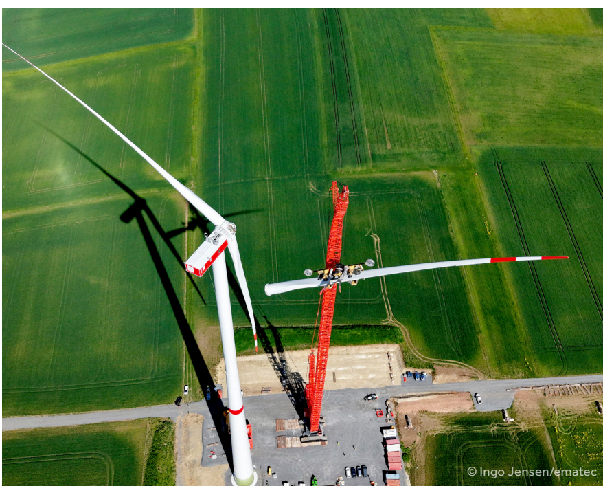
The RBC-D and autonomous positioning system support blade installation where ground access or working space is restricted
