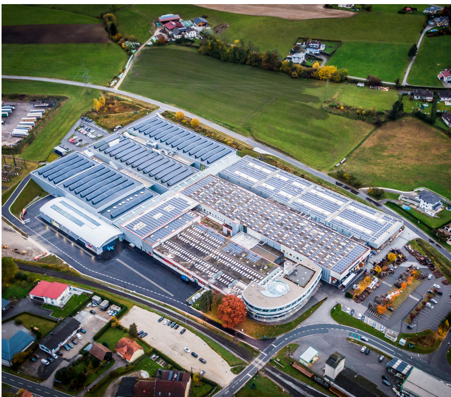
Geislinger production facility in Bad St. Leonhard, Carinthia, Austria
