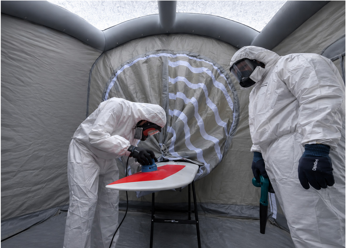
Inside the enclosure, technicians can work in a protected space that separates the repair process from the surrounding environment
