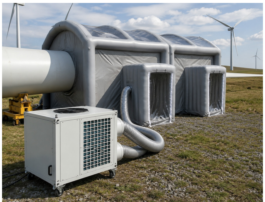
An external heating, ventilation and air conditioning (HVAC) unit can be connected to the enclosure to support more stable temperature and airflow inside the workspace
