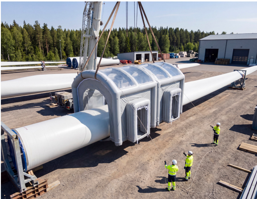
Top installation allows the shelter to be lowered around a selected blade section when access from the tip is not practical
