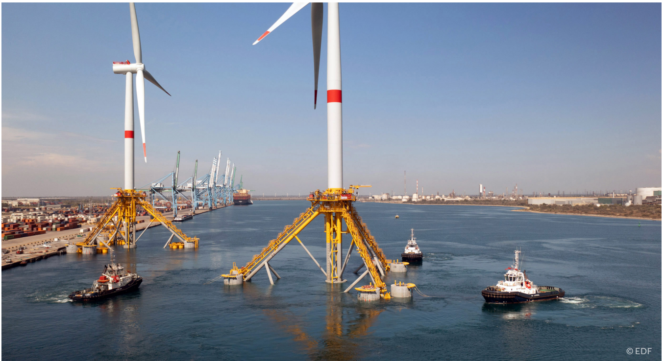
The three wind turbines for the Provence Grand Large project were first assembled on land and in the harbour, and then towed by tugboats to a position 17 km off the French coast
