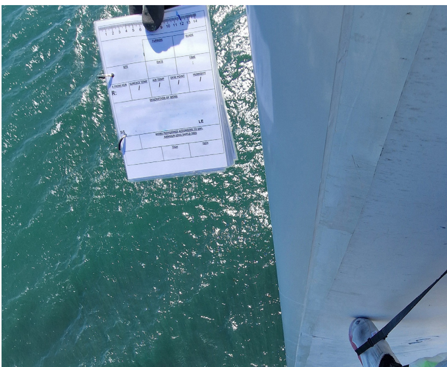
Newly installed Armour Edge LEP
