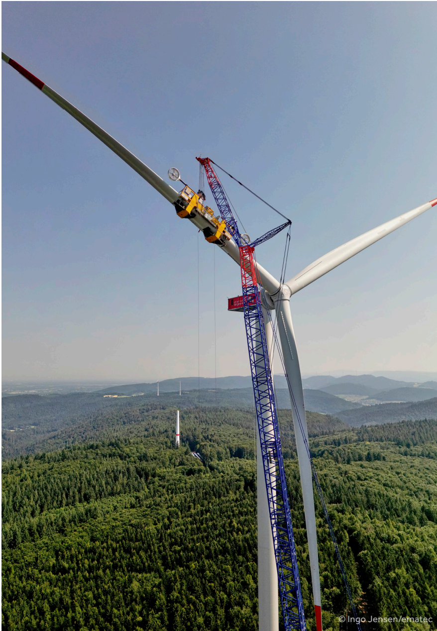
Three new wind turbines from ENERCON are being built at the Schnürbuck wind farm near Ettenheim in Baden-Württemberg with the RBC-D from ematec
