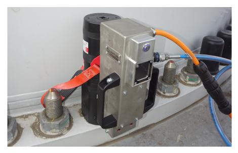
Consider a bolting team using two smart tensioners and two technicians. It takes them three hours to complete an M72 flange before the next tower section can be stacked. With ATR, one technician can remotely oversee multiple robots working in parallel. The next segment can be lifted within an hour. Over five levels, the entire tower could be assembled in a single workday, with robots finishing overnight and collecting them the next morning.
