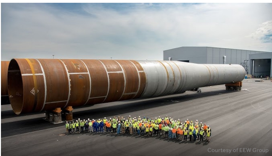
A foundation on a monumental scale: 37 ft (11.3 m) wide at the seabed, supporting the next generation of 12 MW offshore wind turbines at Ocean Wind 1
