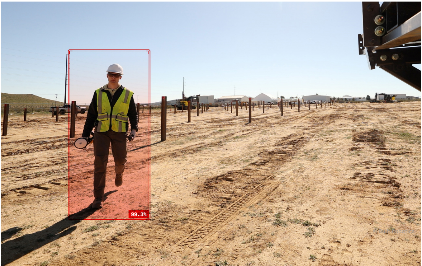
Edge computing processes sensor data locally to support rapid decisions, including detecting people near robots
