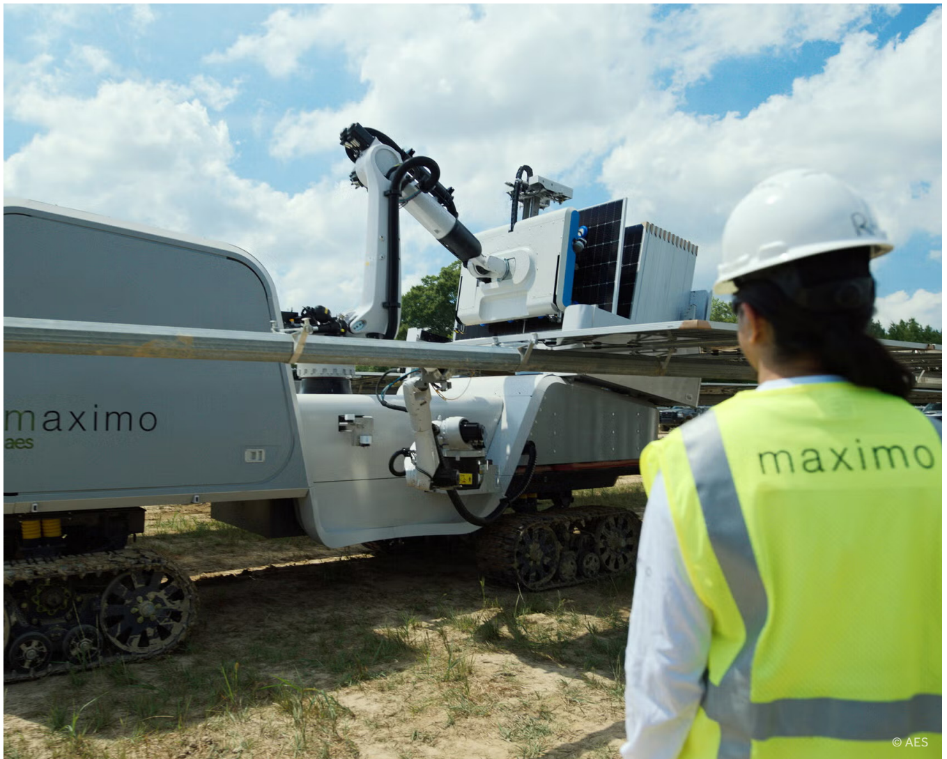
AES's Maximo robot places solar modules onto tracker assemblies
