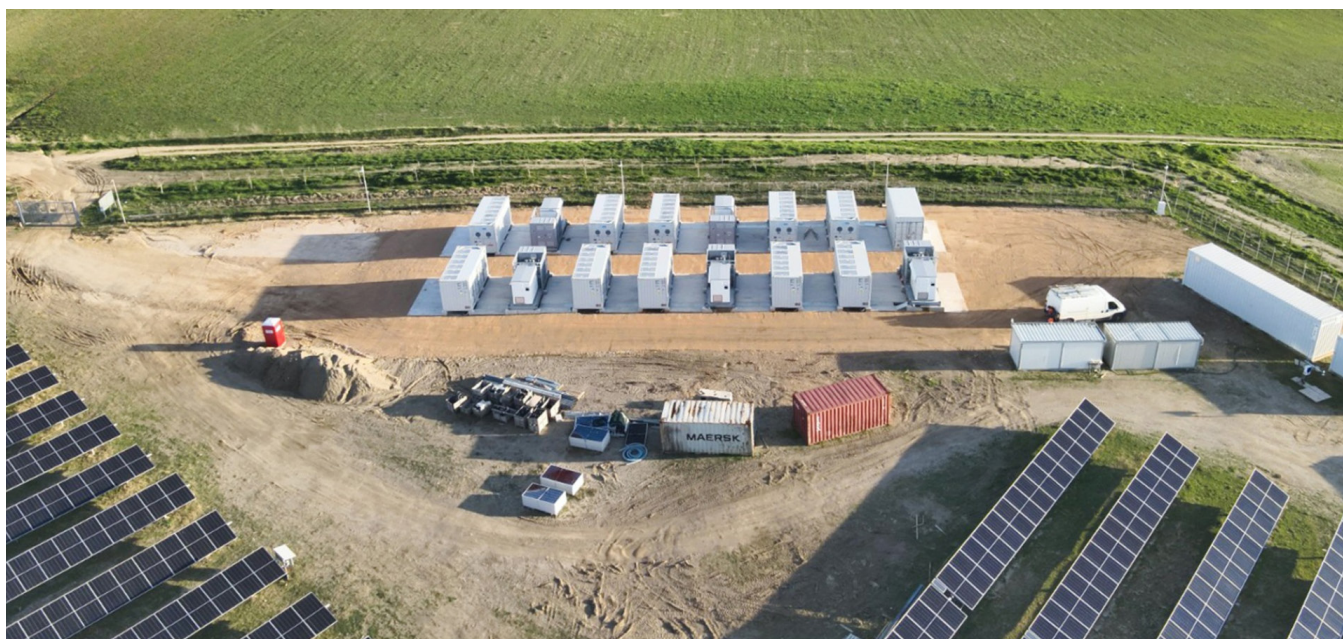
Italy: LONGi's first integrated solar + storage project in Europe
