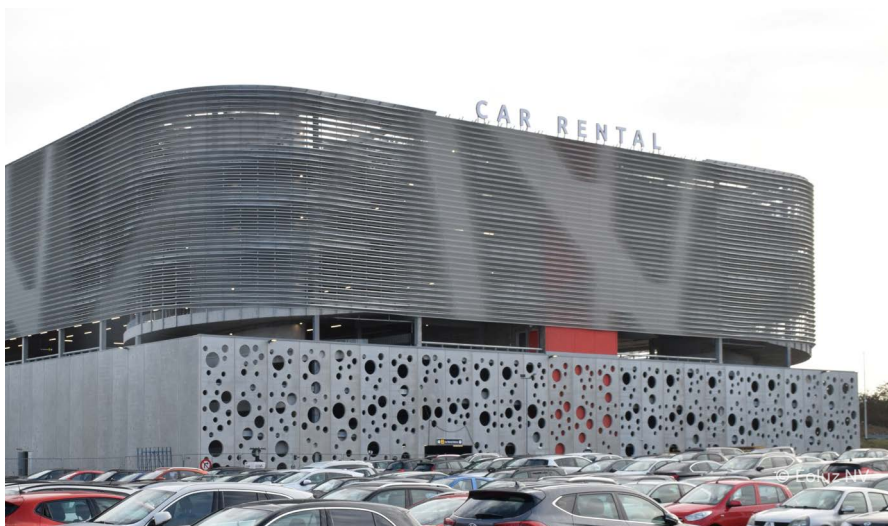
6,000 m 2 of PV modules stretch across the roof of the eight-storey car park of a Belgian airport
