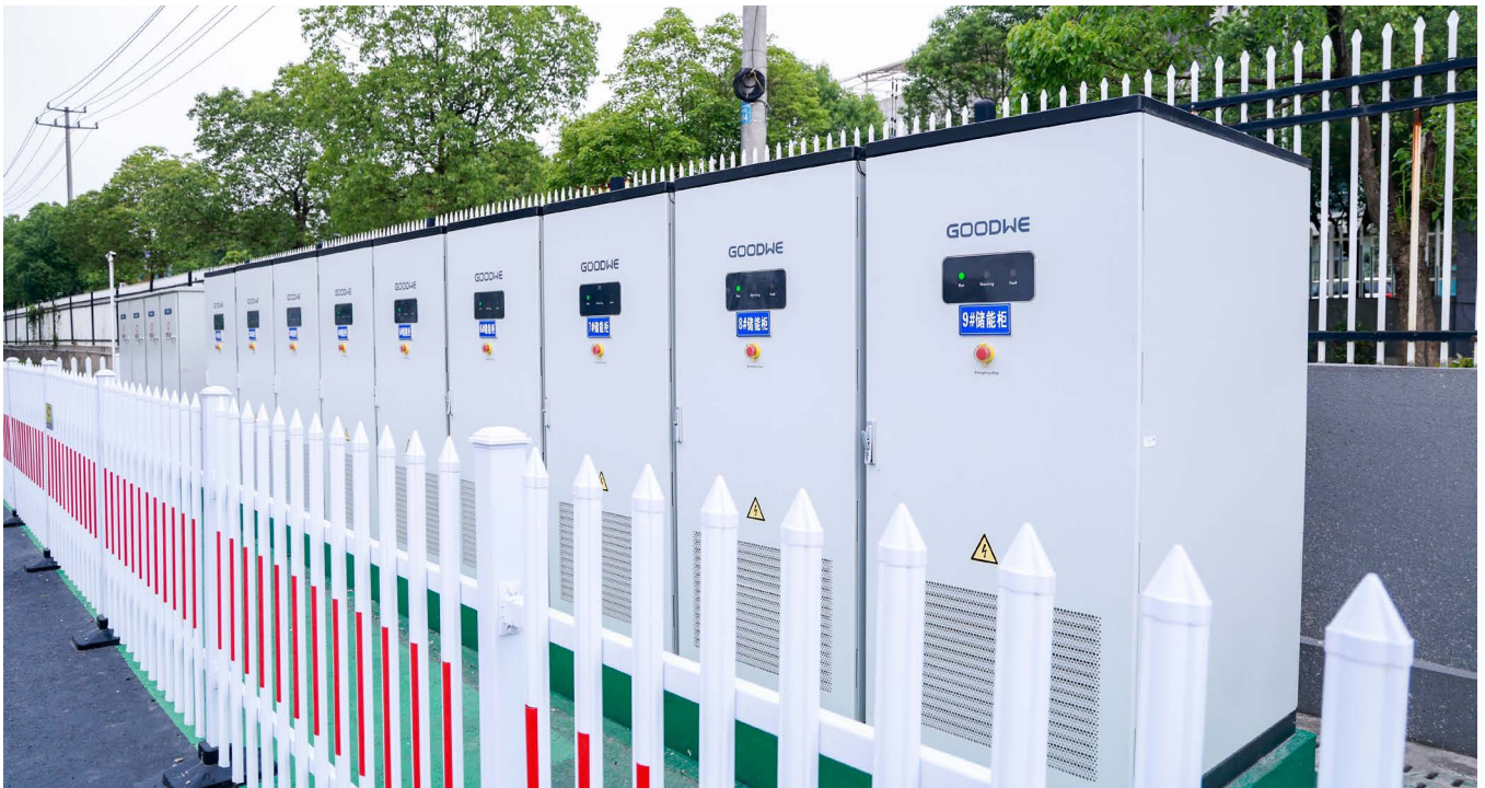
GoodWe has installed nine ESA C&I energy storage systems at their factory in Guangde, China, with 1.125 MW output power and 2.35 MWh storage capacity
