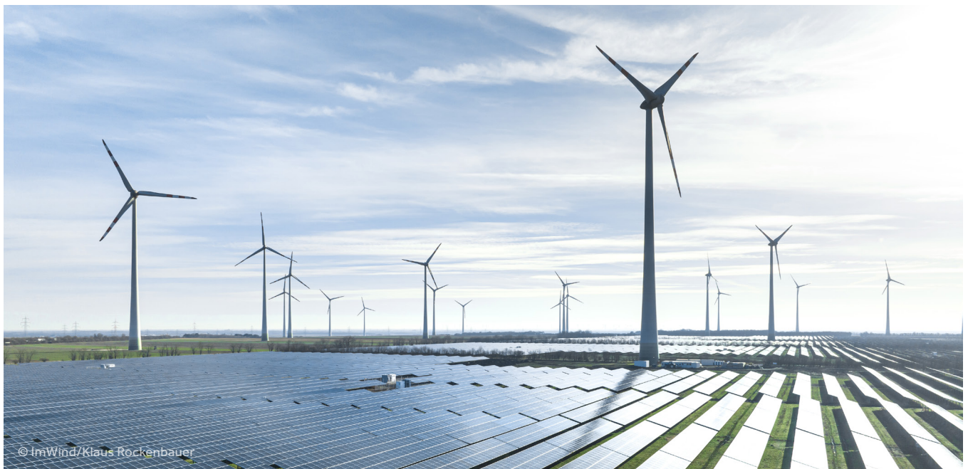
There is a lot of potential in the redensification of existing wind farms with PV
